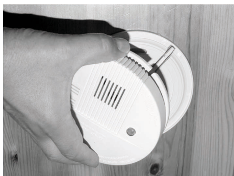
Fig. 205: Removing the housing
