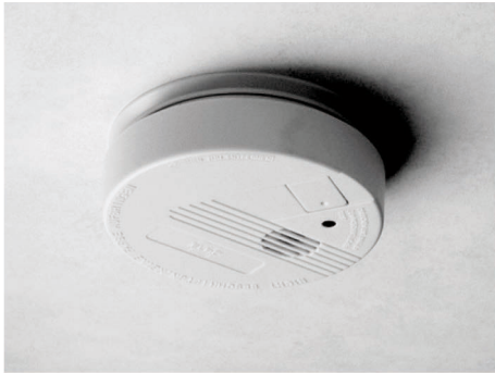
Fig. 43: Smoke detector
