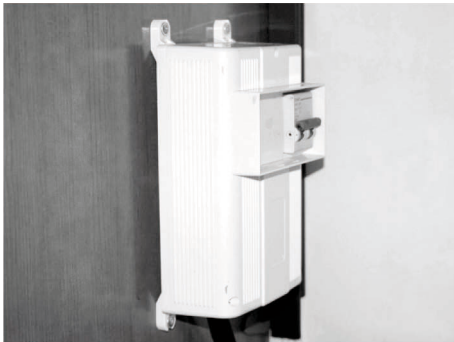
Fig. 3: Ground fault circuit interrupter (GFCI)
