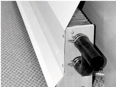
Fig. 83: Convector with thermally conductive panel
