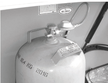
Fig. 71: Gas bottle with low pressure regulator and low pressure hose
