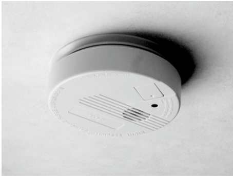
Fig. 39: Smoke detector
