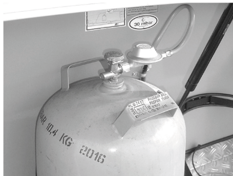
Fig. 64: Gas bottle with low pressure regulator and low pressure hose
