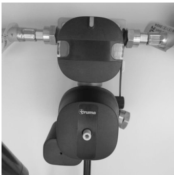
Fig. 114: DuoControl CS gas supply
