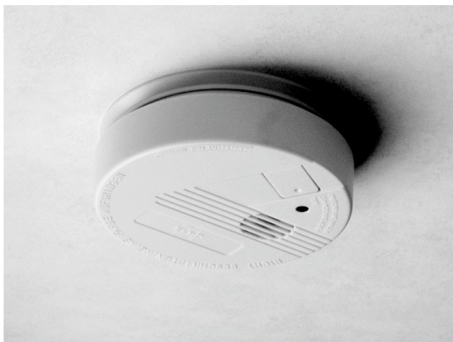
Fig. 59: Smoke detector
