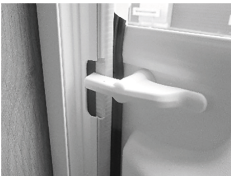
Fig. 33: Door split, locking handle locked
